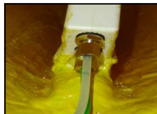
Green and clear pipes connected to skeg box
