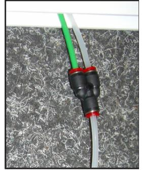
*The two pipes shown connected to the bleed kit drain tube Y piece underneath skeg box*
